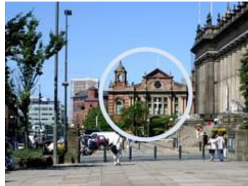
Approaching from the East
